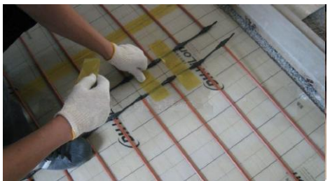
13. Installation of the heating rail
