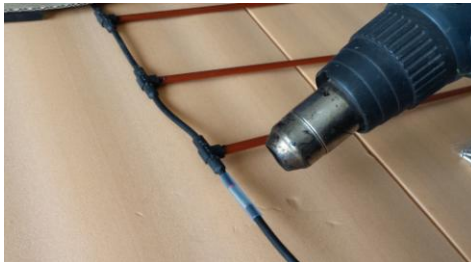
7.Heating the shrinkage tube
